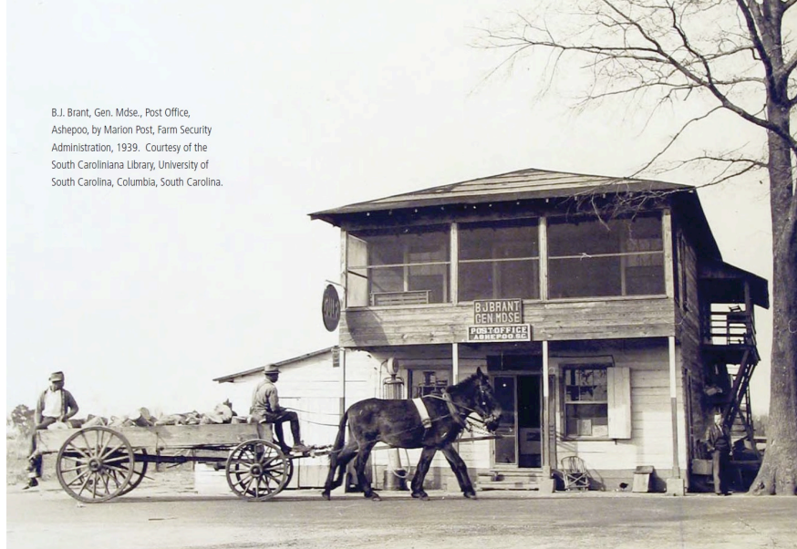
Figure 2: The Exterior of a Country General store in South Carolina
